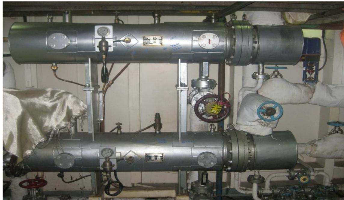
**Fuel steam heating for viscosity control**
